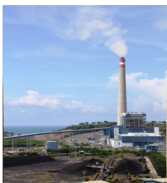
Suralaya Power Plant
